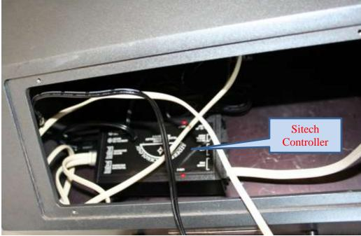
I installed the Az motor assembly (not shown) and reinstalled the bottom plate to the base then connected the Controller to the Az motor and used Velcro to attach it to the inside Base plate.
